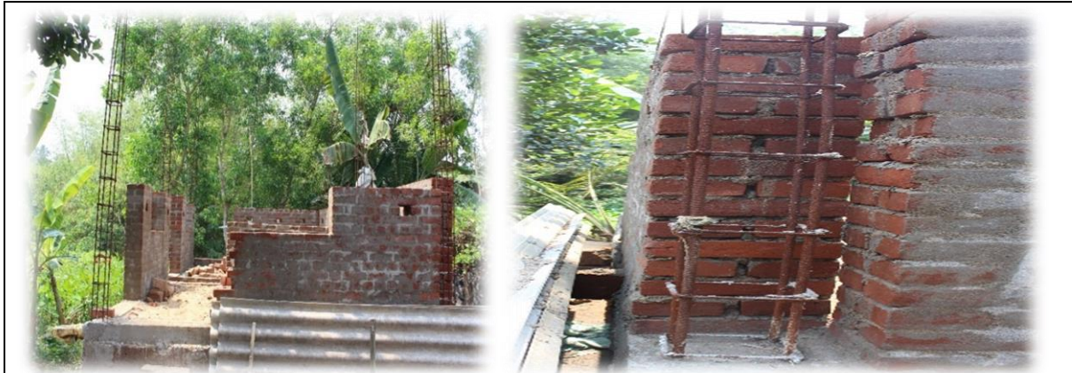
Use of steel rod for construction of PMAY-G house as per the design suggested
